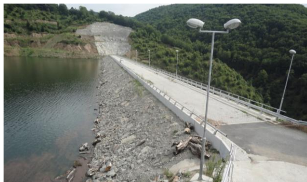
Fig. 12. Rock-fill dam Knezevo with asphalt core, on river Zletovska, built in 2011, H_s=82 m
