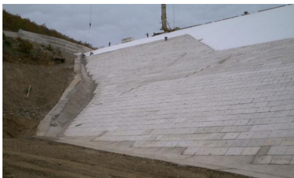
Fig. 11. Rock-fill dam Loshana with geomembrane facing, built in 2006, H_s=45 m
