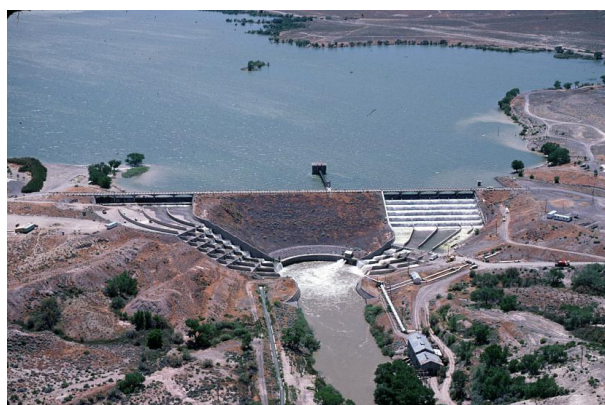
Slika 4.5 Kombinovani prelivi Lahontan brane, reka Carson, Nevada USA
